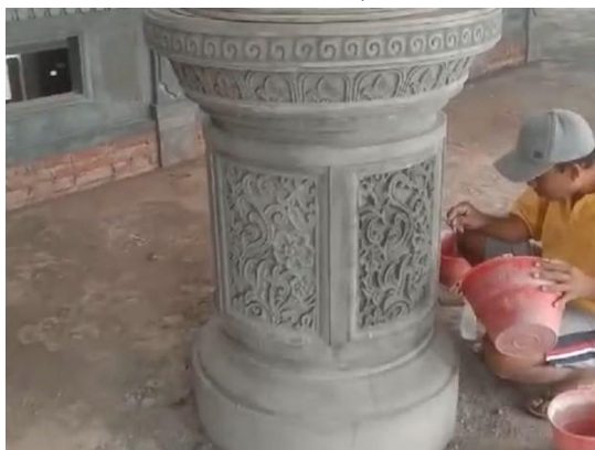
Figure 6. Process of Making the Pillars of the Jami' Nurul Hayat Mosque Adopting Balinese Ornaments
