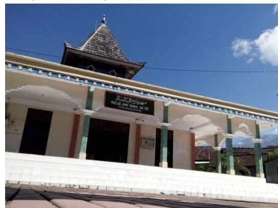
Figure 7. Exterior view of the Jami' Nurul Hayat Mosque
